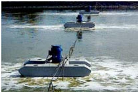
process falls short. While this lack of efficiency can be overcome somewhat by employing more aerators, these added aerators increase the operating costs and the potential for downtime. In any event using more aerators of poor performance is not a practical solution.
