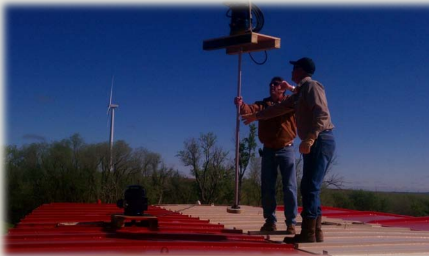
Installing turbine aerator into a frac tank.
